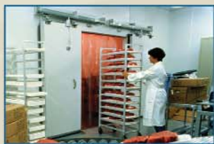
Inside walk-in coolers
