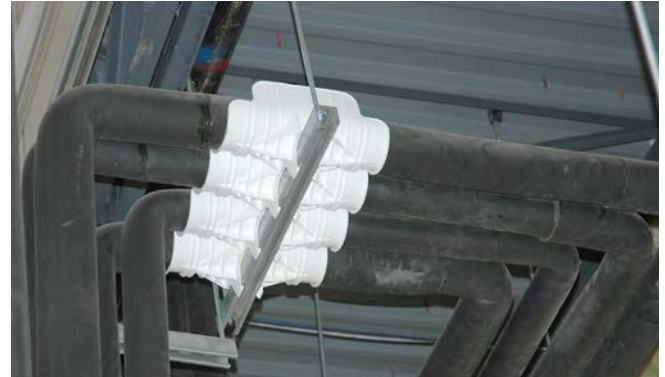
Ceiling Run with Supports
