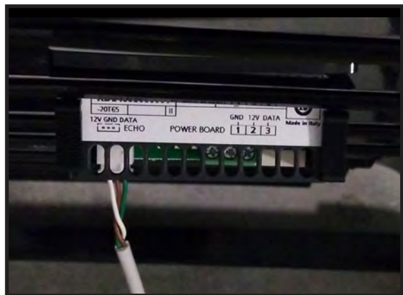
Rear of Control
