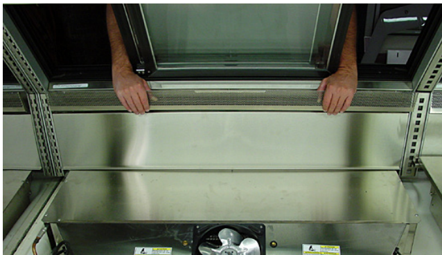
STEP 7 – Lift out discharge air grille.
