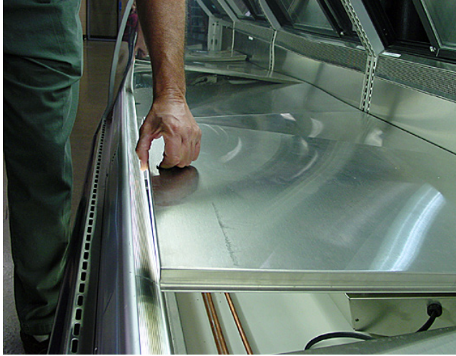
STEP 6 – Lift out display pan support.
