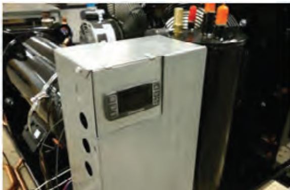
Figure 10 – Silver Electrical Box
