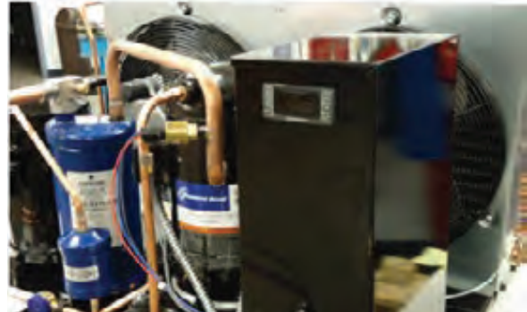
Figure 12 – Large Black Electrical Box
