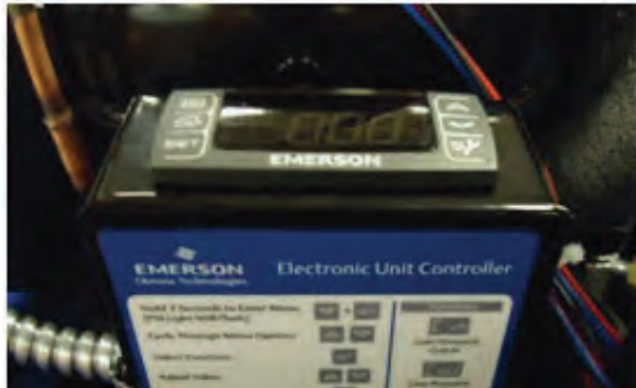
Figure 11 – Small Black Electrical Box
