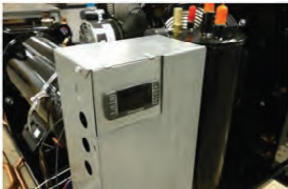
Figure 10 – Silver Electrical Box
