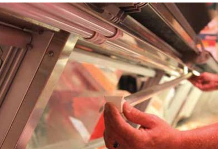
**Hussmann's EcoShine Quick Connect LED can be installed by simply replacing ballasts and inserting the new LED into the existing fixture.**
