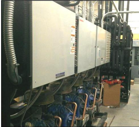
**Hussmann's TerraChill CO<sub>2</sub> system reduces HFC refrigerant charge by more than 65%, resulting in a positive impact on Hy-Vee's carbon footprint.**
