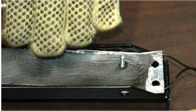
Gasket starts from below holes on top of the mullion as shown
