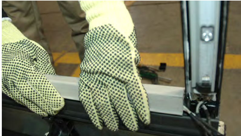
Bottom Rail Retainer
