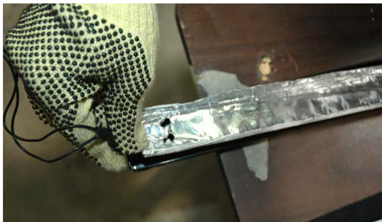
Replacement Heater in Mullion
