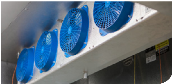
Shown: Krack KR Series Compact Unit Cooler for Freezer Applications
