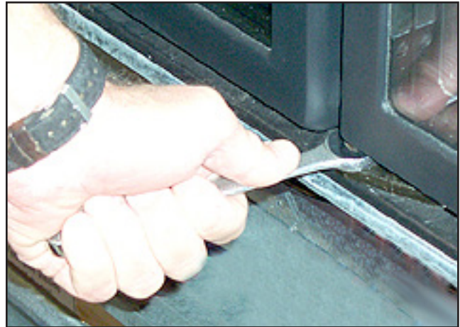
Adjust Closing Torque
