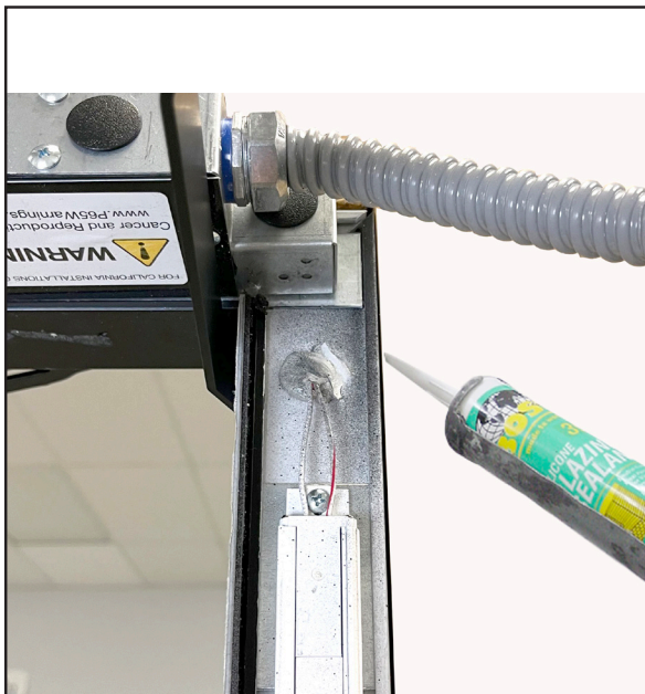
Apply Silicone Around Frame
