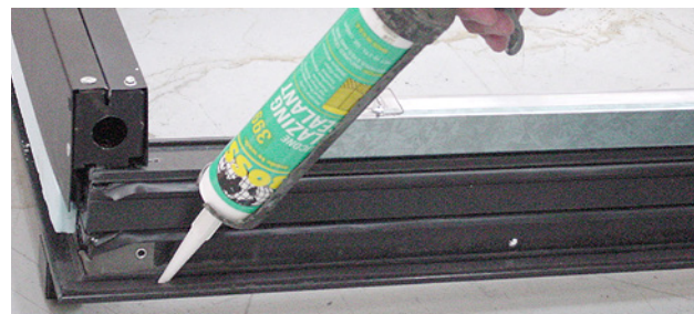
Apply Silicone Sealant
