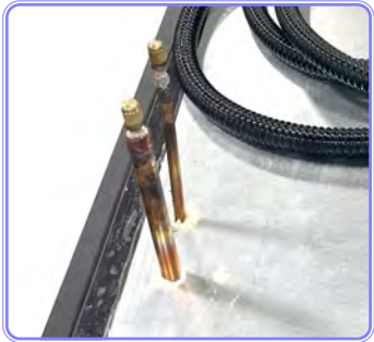
Seal piping penetration on top of case.
