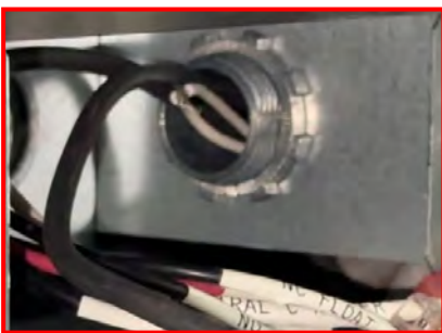
(Step 2) Pass wiring through conduit.
