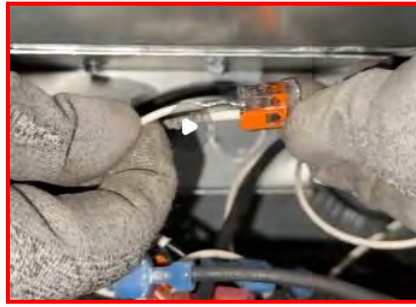
(Step 4) Condensate Heater No Float Switch Connection
