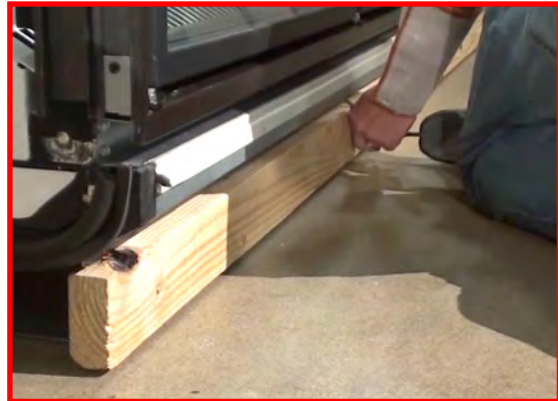
Remove Front Shipping Brace
