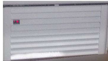
Lift up and out to remove access panel
