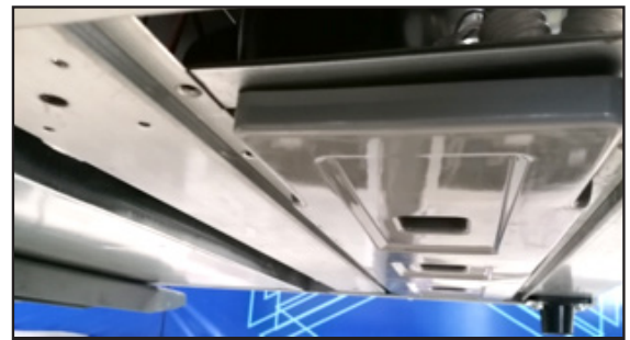
Condensate Pan Installed
