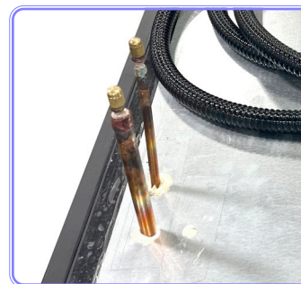
Seal piping penetration on top of case.
