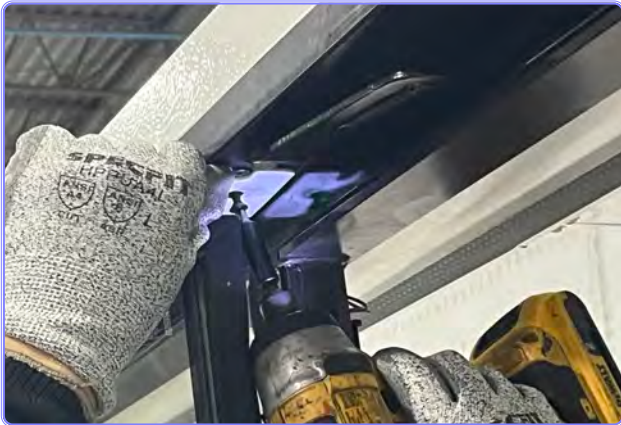
Slide torsion pin up and onto frame pin.
