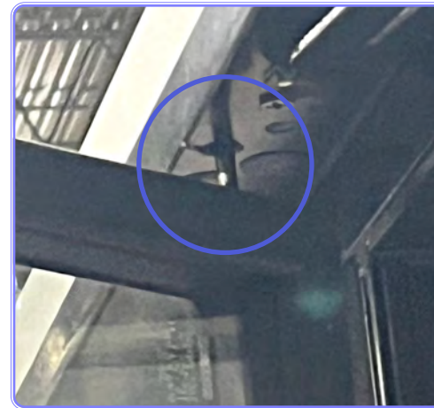
Slide torsion pin up and onto frame pin.
