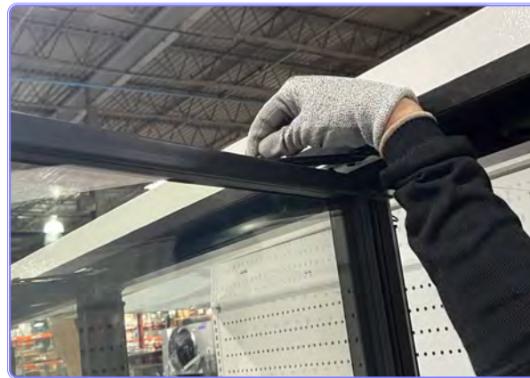
Install door cam at top of door.
