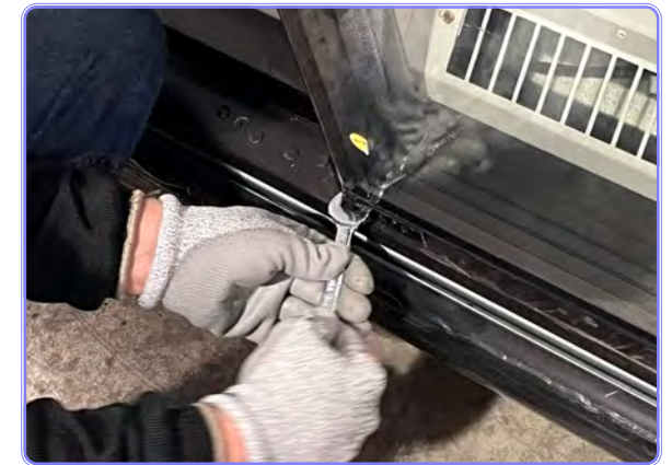
Slide torsion pin up and onto frame pin.
