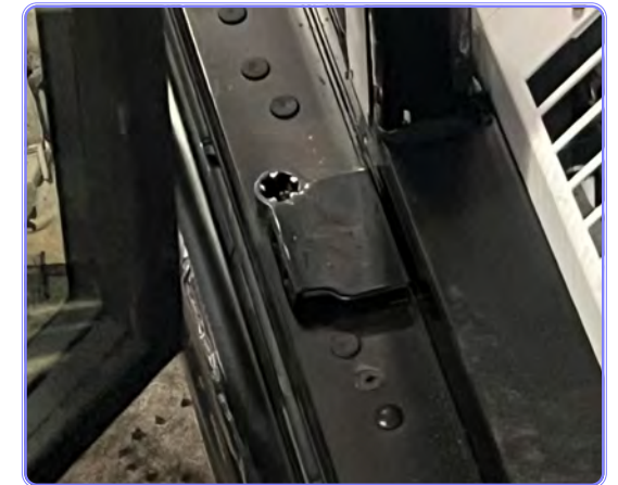
Door removed from bottom of torsion plate.
