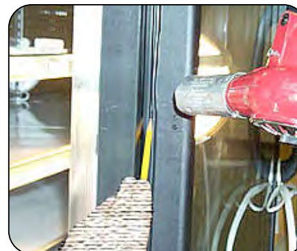
Pulling Gasket Into Place With a Pencil
