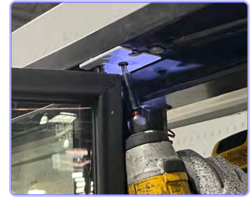
Remove screw from door retaining plate
