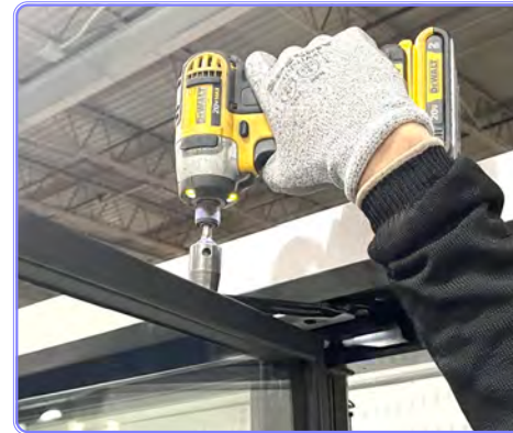
Remove door cam from top of door(s).
