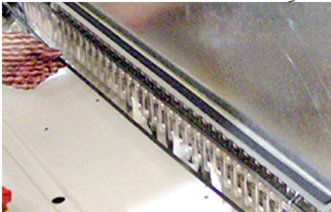
Clips to be located 5-6 inches from bracket
