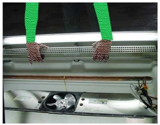
STEP 12 – Rotate fan plenum up and back; hook chain at rear of liner.
