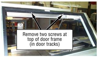
5. Pull back the top of the door frame approximately 2 inches. This will allow clearance for removal of the stainless steel top liner and trim pieces.
