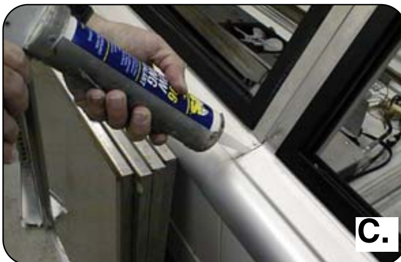
Figure 16. Sealing Case Joints
