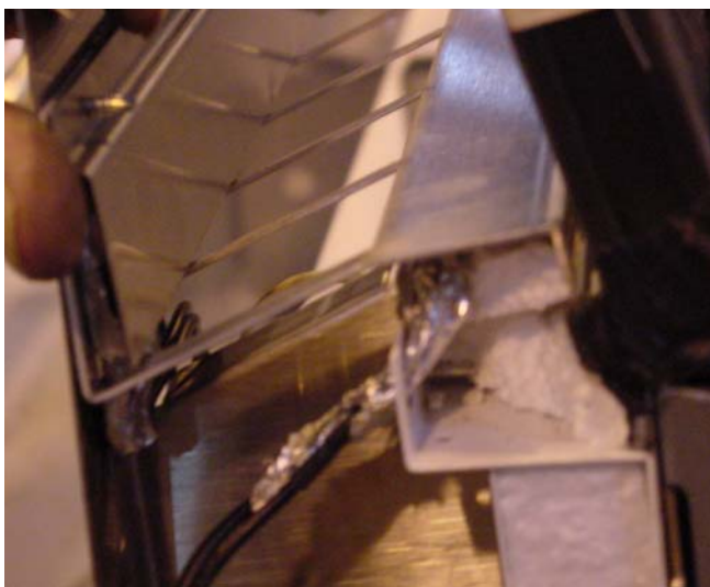
Detail Shows Wiring in Place, with Return Grille Installed.
