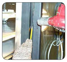
Figure 15. Pulling Gasket Into Place With a Pencil
