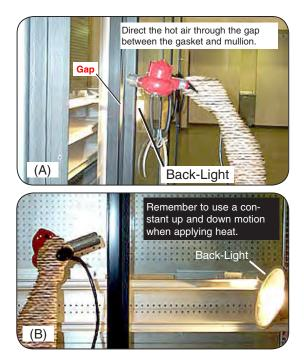
Figure 13. Applying Heat to Gasket
