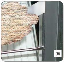
Figure 17. Removing Door Wireway Covers
