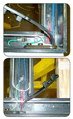
Figure 18. Replacing Door Frame Heaters
