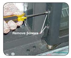
Figure 4. Removing Screws to Plug
