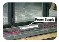
Figure 22. Power Supply Location
