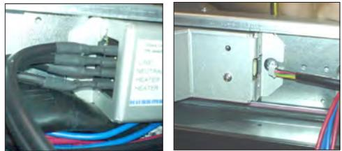
1. Remove the mullion cover between the pair of doors where the sensor is located.
