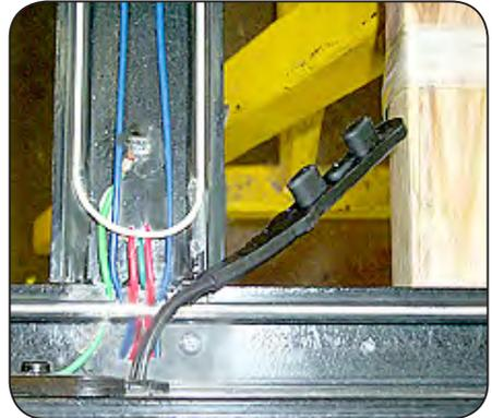
Figure 18. Replacing Door Frame Heaters
