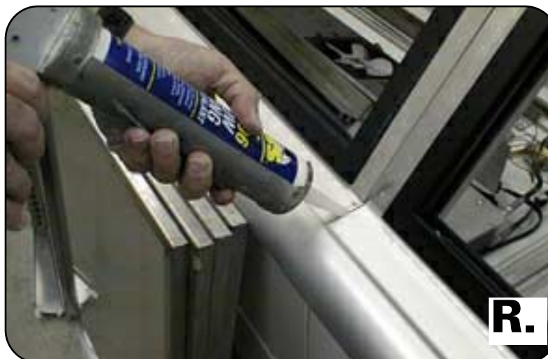
Figure 14. Sealing Case Joints
