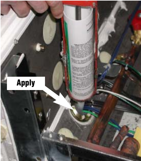
Figure 17 — Seal Electrical Nipple
