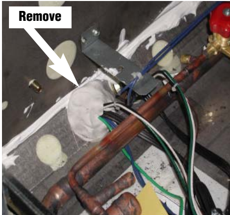
Figure 12 — Remove Sealant
