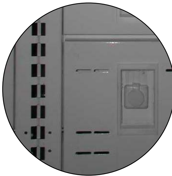
Socket with Cap Installed
