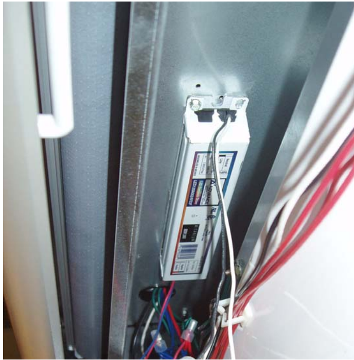
Figure 5 — Install Power Supply
