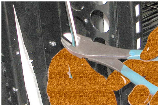
Figure 10A — Cut Power Wires
