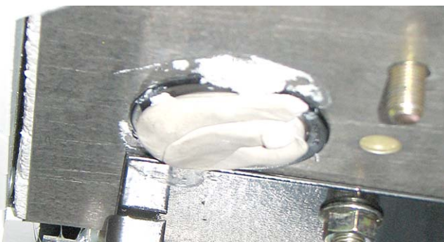
Figure 13 — Plug Conduit with Permagem
