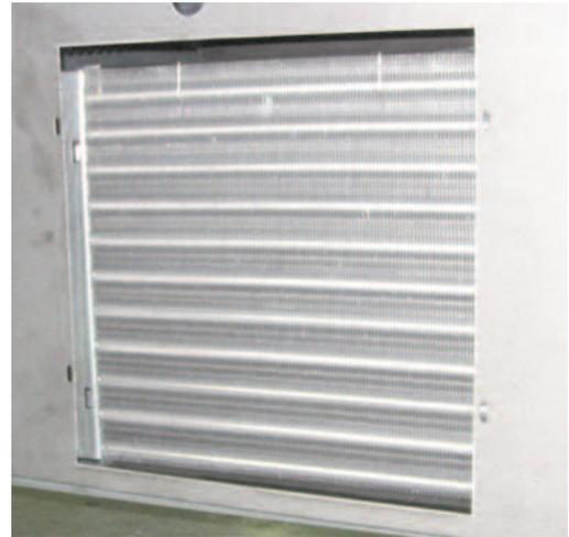
Airflow blockage increases energy consumption and reduces the merchandiser's ability to maintain operating temperature.
