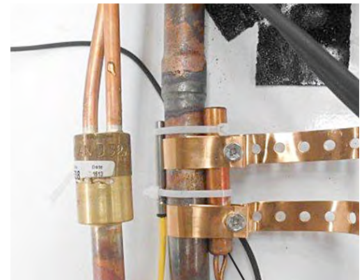
Defrost Termination Sensor
