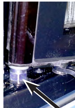
Not Properly Engaged in Hinge Plate
