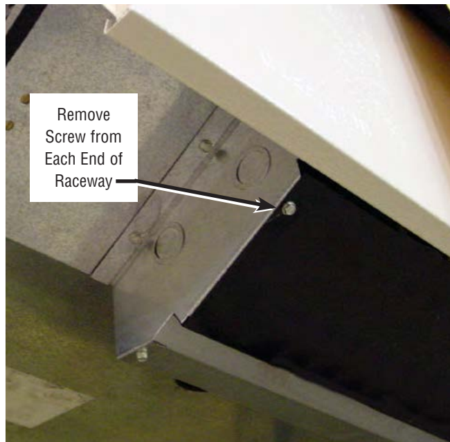
Raceway Access at Left Hand End
