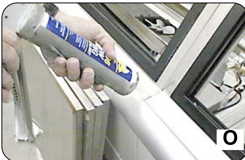
Figure 13. Seal Case Joints
