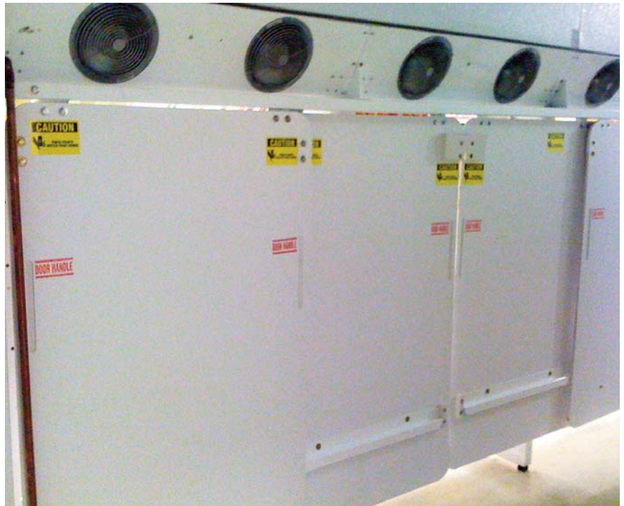
Rear Sliding Doors Installed in Rear Roll-In Display
