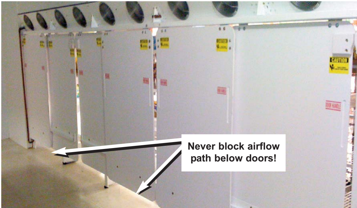
Rear Sliding Doors Installed in Rear Roll-In Displays
