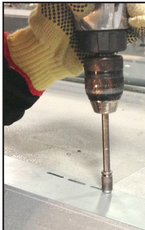
Figure 20-1 Fasten Canopy Fascia
