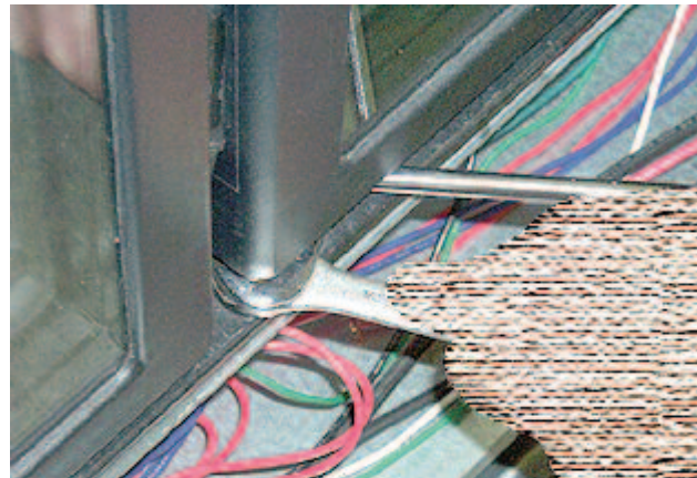
Figure 1. Adjusting Closing Torque
