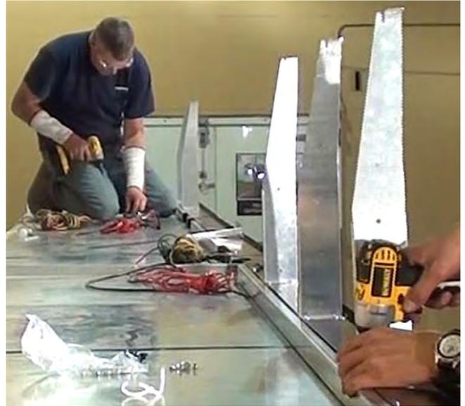
**Install Facade Supports using holes provided**
