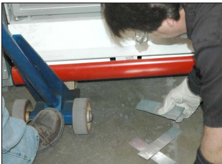
Figure 7: Level Cases with Shims
