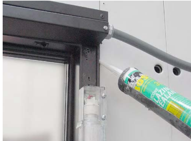
Apply Silicone Around Frame
