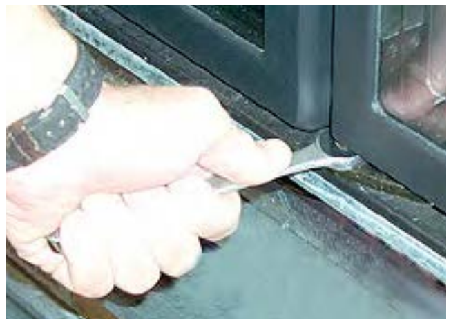
Adjust Closing Torque
