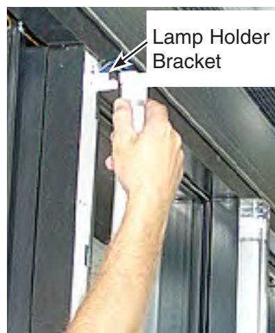
Remove Lamp Holder from Bracket
