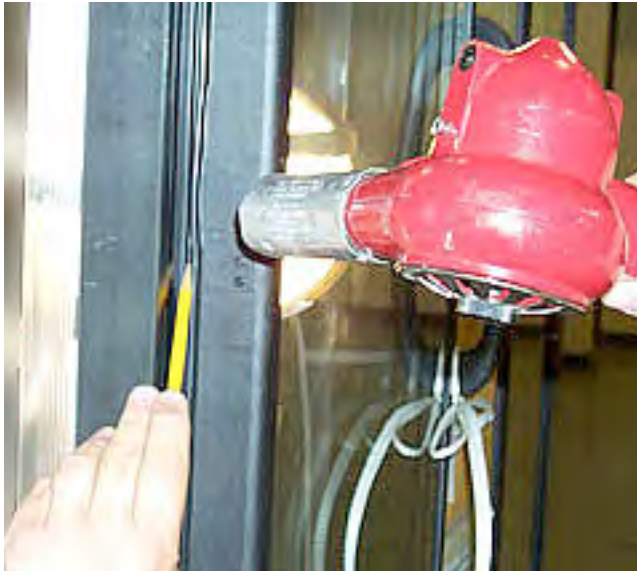
Pulling Gasket Into Place With a Pencil
