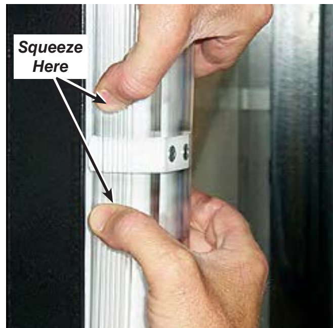
Disengage Diffuser Clips
