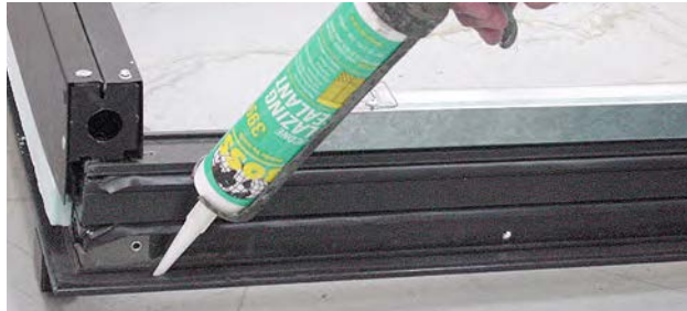
Apply Silicone Sealant
