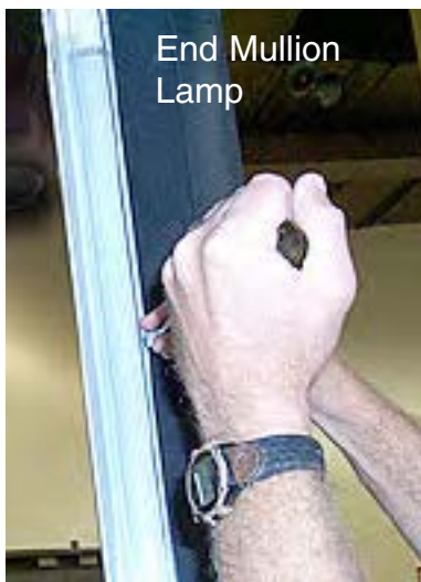
Remove Diffuser from End Mullion Lamp
