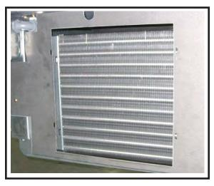
Airflow blockage increases energy consumption and reduces the merchandiser's ability to maintain operating temperature.
