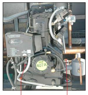
Remove bolts from Copressor Housing
