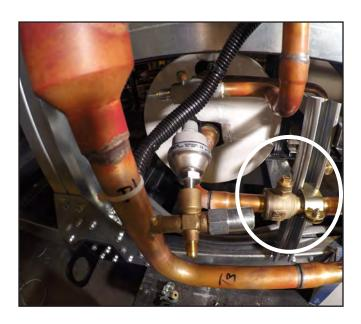
2. Close the ball valve at the inlet to the receiver pressure regulating valve
