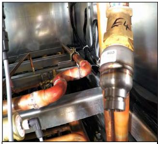
ELECTRONIC EVAPORATOR PRESSURE REGULATING VALVE (EEPR)
