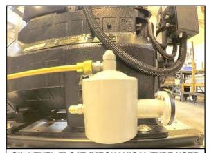
OIL LEVEL FLOAT (MECHANICAL TYPE USED ON MEDIUM TEMP RECIP COMPRESSORS
