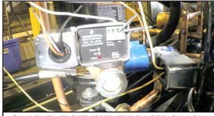
OIL LEVEL FLOAT (OMB TYPE USED ON LOW TEMP SCROLL COMPRESSORS
