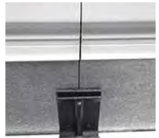
Install case-to-case joining brackets
