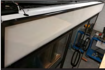
Display Slides out to access Wireway
