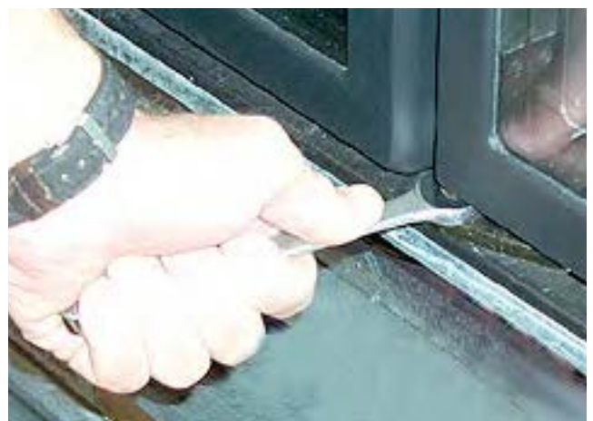
Adjust Closing Torque
