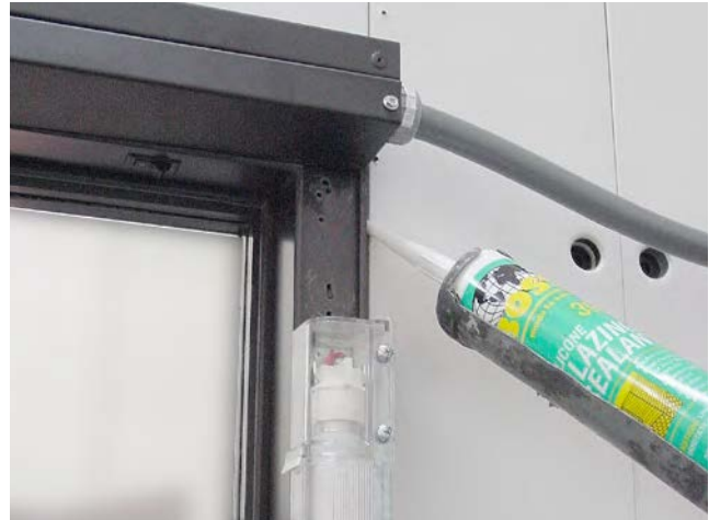
Apply Silicone Around Frame
