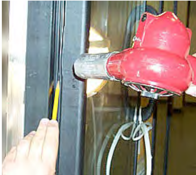
Pulling Gasket Into Place With a Pencil
