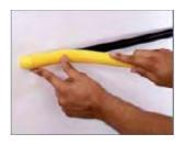
2a. Flexible Top: Butt end of the vinyl top against end/corner cap. While applying pressure, bend back vinyl top so that vinyl legs are positioned within the base grooves. Roll vinyl top over full length of base, then tap with rubber mallet to ensure vinyl is securely locked into the base. 2b. Rigid Top: Snap the Rigid Top over the Rigid Base.
