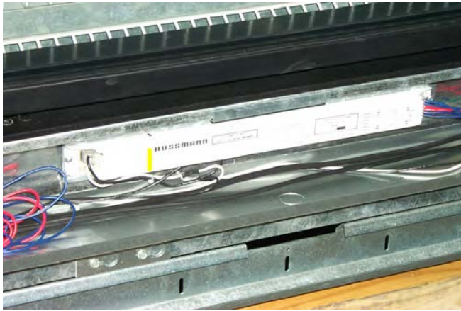
Remove Ballast & Install Power Supply (Typical Installation)
