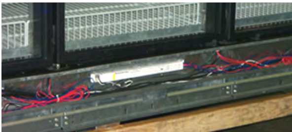
Remove Panels to Locate Ballast (Typical Installation)
