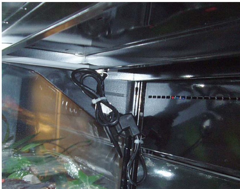
Figure 11 — Contain Excess Wire
