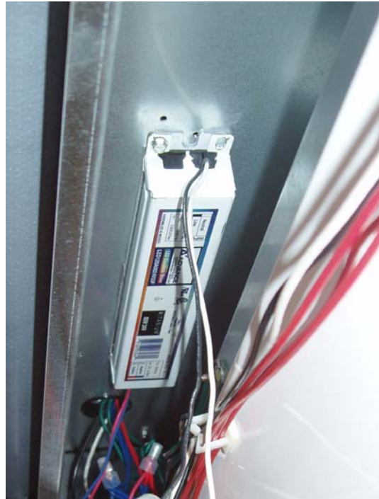
Figure 5 — Install Power Supply
