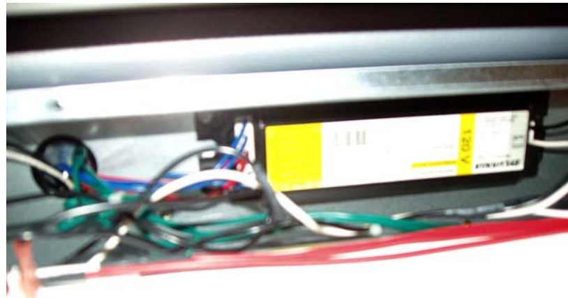
Figure 5 — Remove Shelf Lamp Ballast
