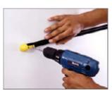
Attach the base and end/corner cap to the desired surface by inserting #8 pan head screws through the pre-slotted holes in both the end cap and the base. Insert screws through the two holes of end cap and tighten.
