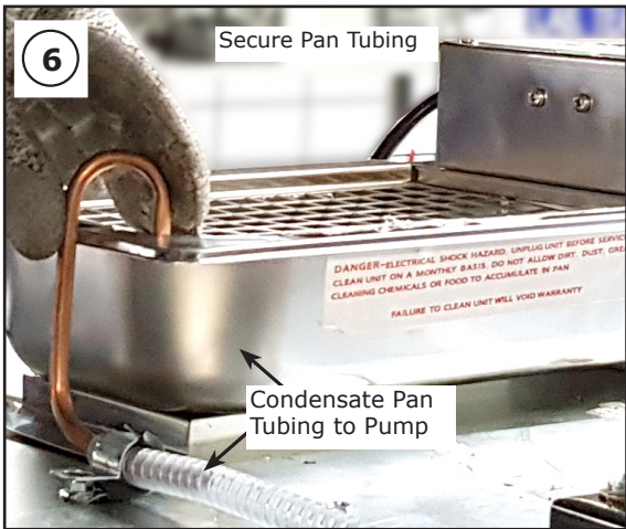
Condensate Pan (Installed on top of case)
