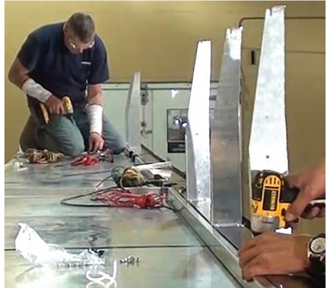
Install Facade Supports using holes provided
