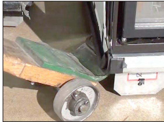
Use J-Bar to Align Cases for Joining
